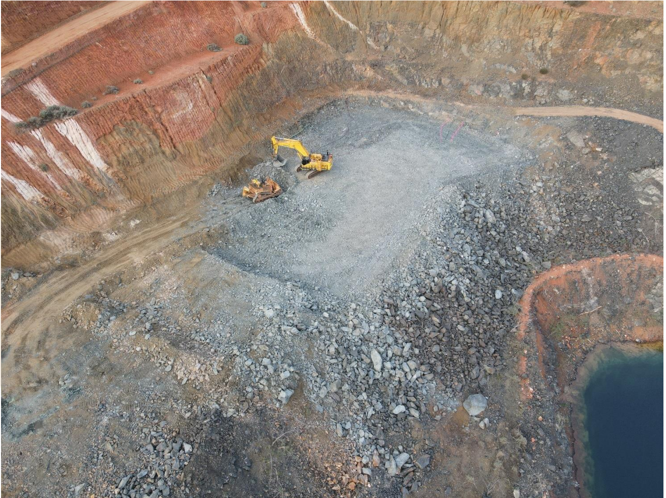
Establishing working area, bunds and pit floor at Missouri
